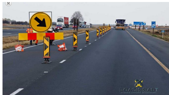
Figure 3 - One lane closed due to construction and traffic flow is managed.
